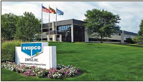
EVAPCO Global Headquarters, Taneytown, Maryland USA
