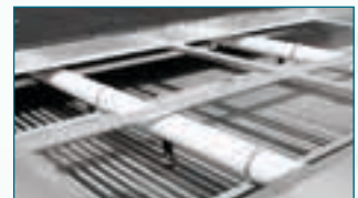
Drift Eliminators Removed for Coil Inspection
